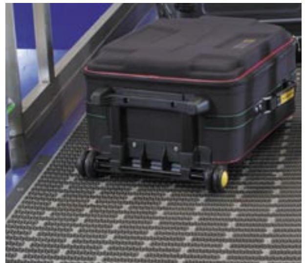
Airport baggage handling conveyor
